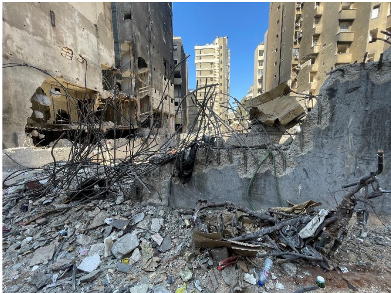
Damage caused by an airstrike in Beirut © Action Against Hunger
