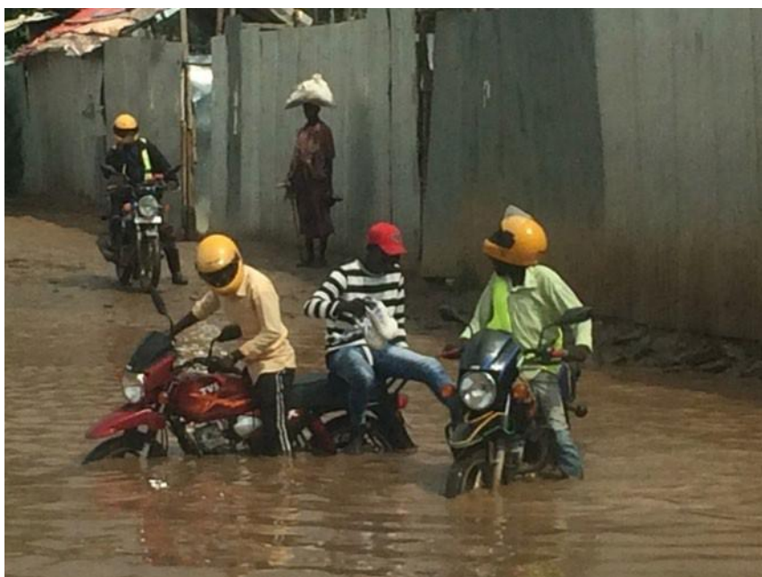
Figure 11: The road network is of poor-quality inhibiting movement around the camp particularly after rains. Photo Credit: JRS
